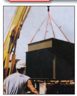
Adjustable Rope Slings replace multiple, "non-adjustable" slings by accommodating a range of dimensional requirements with infinite adjustability.
